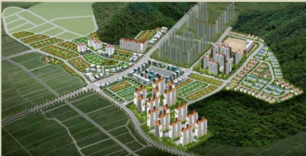
Project Name: Boolro complex land readjustment project (2 division) Location: A1 district, Boolro complex 2 division, Incheon Area: 43,000m 2
