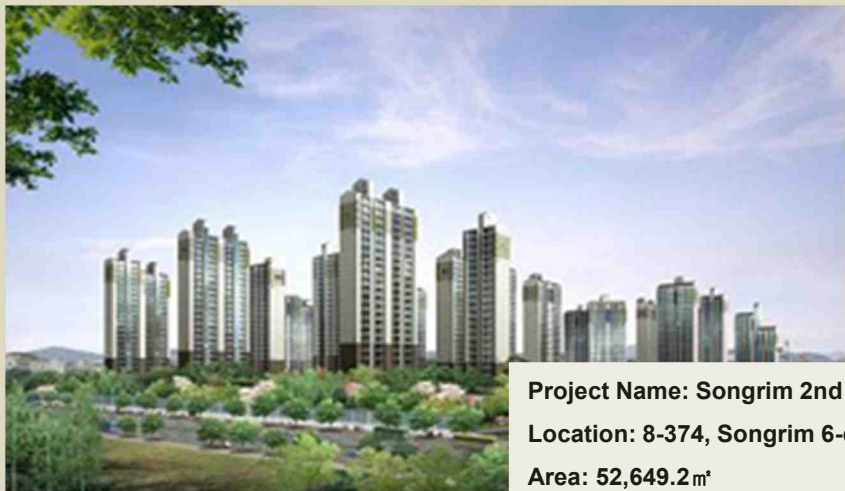
Project Name: Jugong Apt. reconstruction project in Shinhyun-dong Location: 3 district beside 254, Shinhyun-dong, Seo-gu, Incheon Area: 163,872.70m 2 Size: 3,331 households
